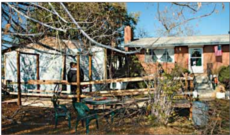
Students in Mike Greeley's Building Construction class erected a 50-foot wheelchair ramp at Jonathan Page's home.
